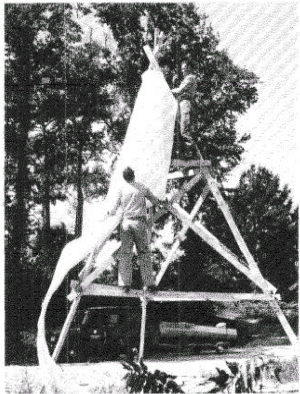
FIGURE 3 - 5. Construction of a large tripod signal
